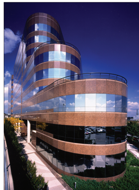
Forchelli Deegan Terrana LLP office, top floor of the OMNI building
